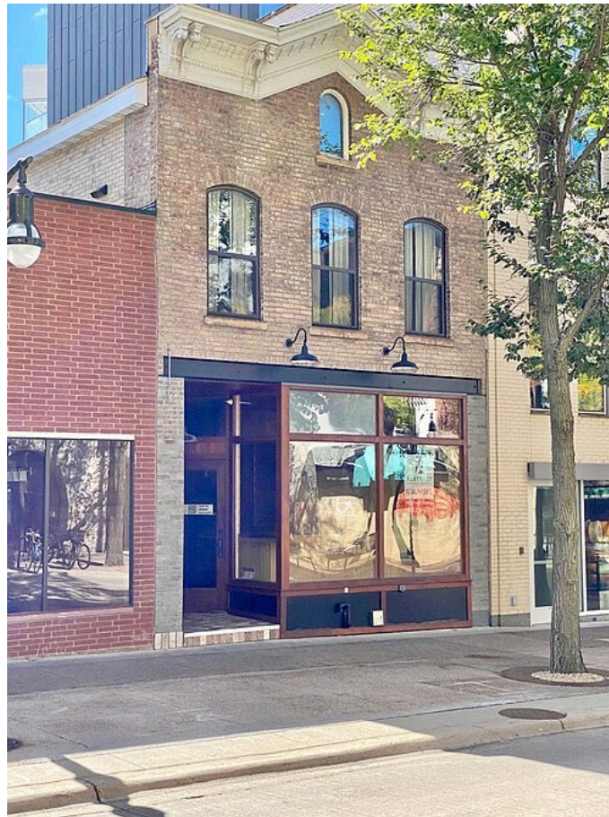
Figure 4-1 Original Cornice on Historic Masonry Building
