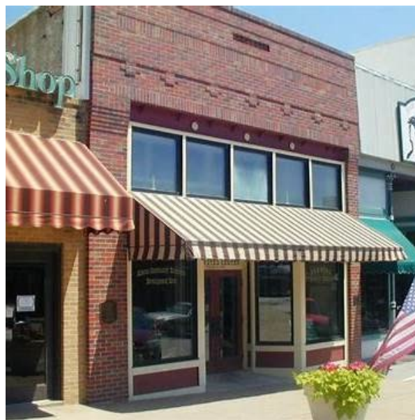
Figure 7-1 Awnings and Canopies
